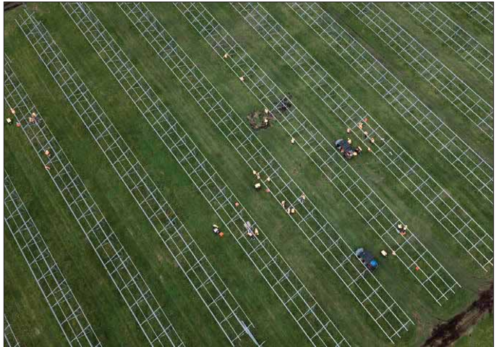
An aerial view of rows of solar panel piles at Ruakākā
