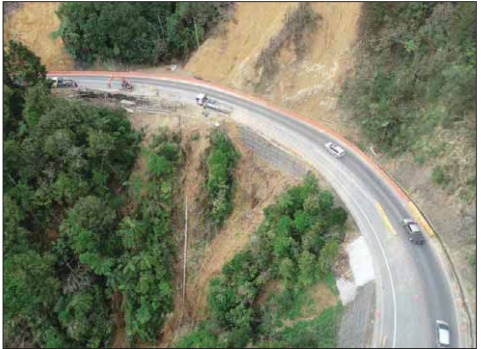
Major slips developed on the Brynderwyn section of State Highway One when Cyclone Gabrielle arrived in Northland in February 2023
