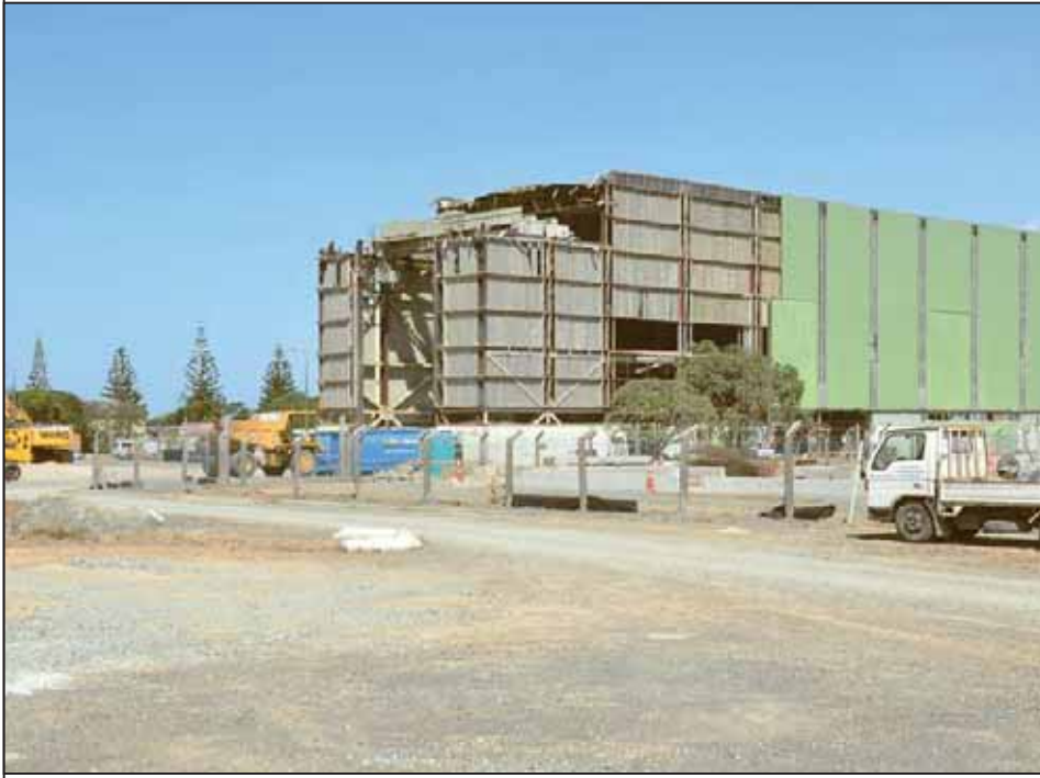
Dismantling of the Marsden A Power station has recommenced after a halt to accommodate the fish spawning season at the NIWA aquaculture plant alongside.
