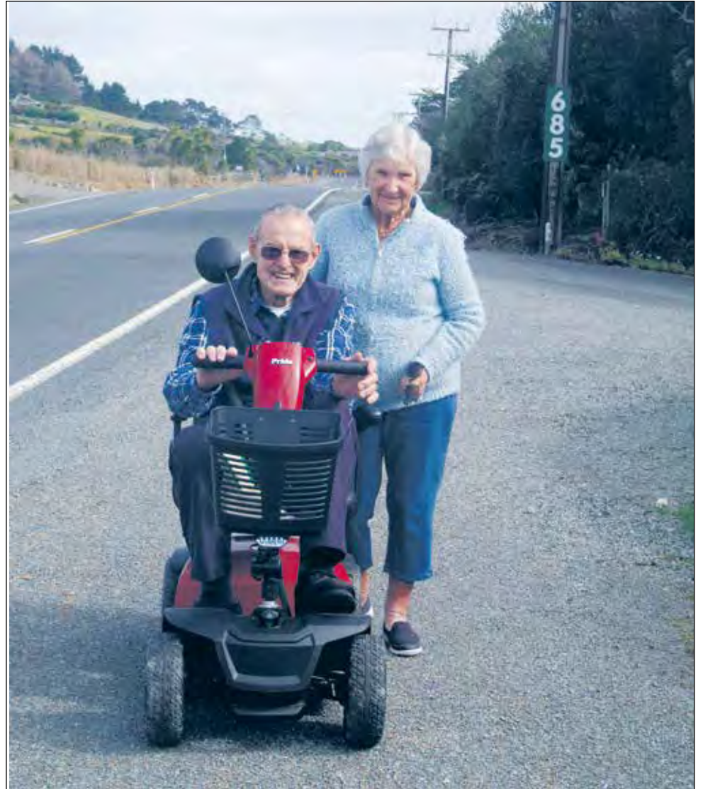
Cynthia and Roy Voss are enjoying the new section of the Waipu Cycle and Walkway under construction at Waipu Cove
