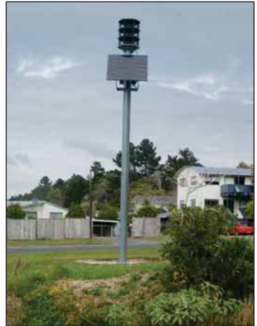
New solar powered tsunami sirens are being progressively installed around Northland but it will be the old sirens that get tested at 10am on Sunday 29 October at the beginning of daylight saving. Above: the Ruakākā Village's new siren.
