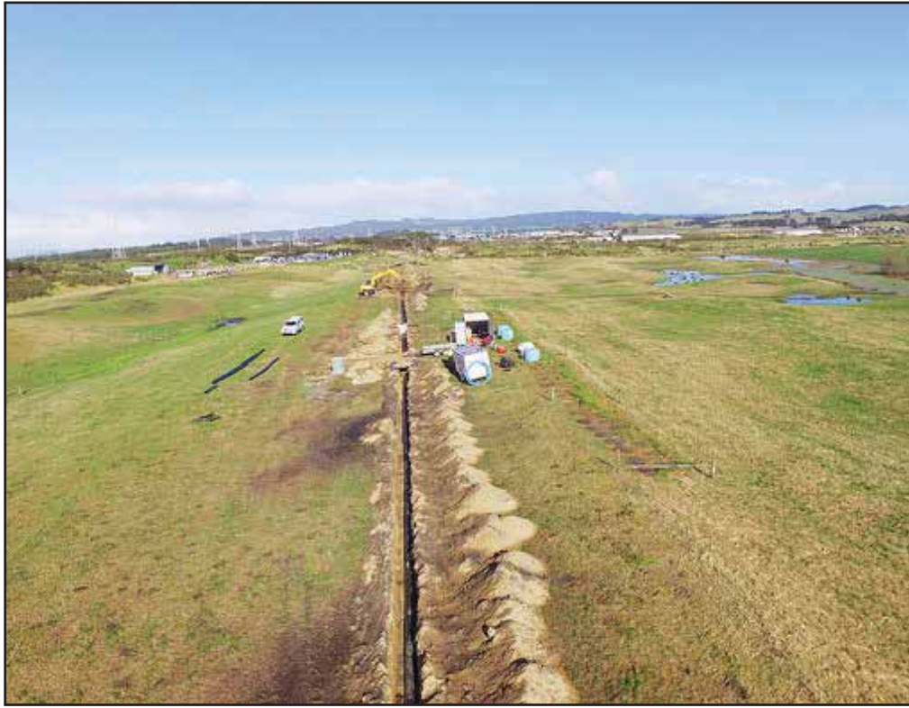
The new pipeline taking treated wastewater to the Rama Rd. disposal field was installed in July.
