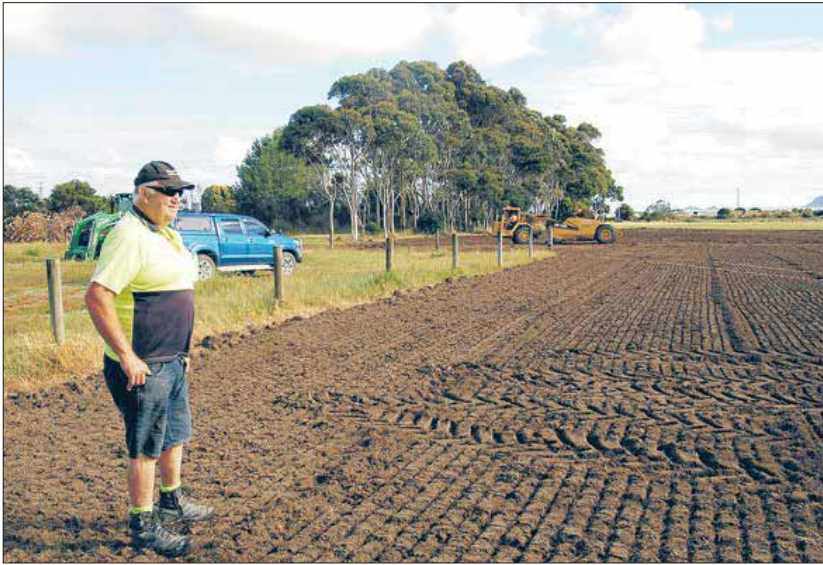
Tony Jelas as work sorting the drainage at the Ruakaka sports fields
