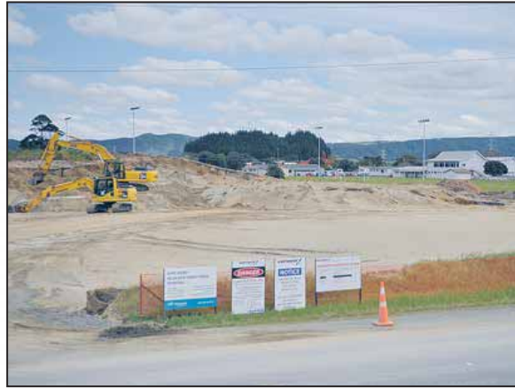
Ruakaka sports park sand ridge is being removed to make way for new sports fields
