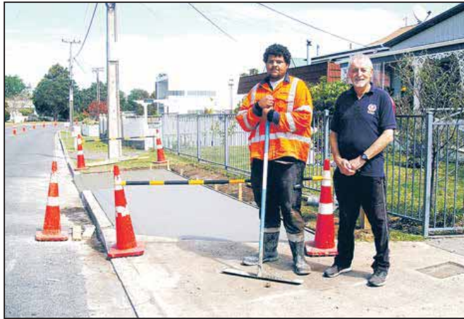
Ruakaka Residents and Ratepayers Association Chairman Jules Flight inspects a section of the new footpath with Erik Tali of Downers. Mr. Flight said One Tree Point people have been asking for a footpath for the 30 years he has lived in the area and probably for longer than that.
