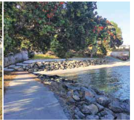
Paradise Point seawall
