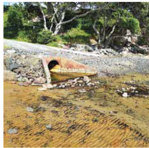
Rock revetment, SW and accessway
