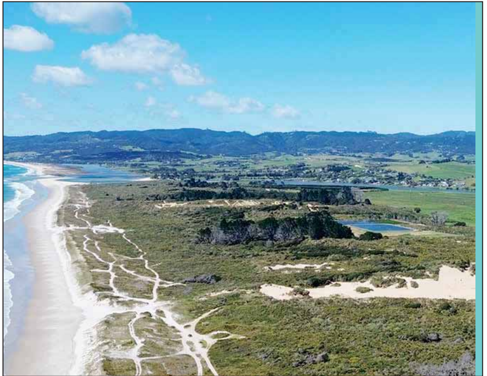
The Waipu wastewater treatment ponds in the dunes north of the Waipu Estuary
