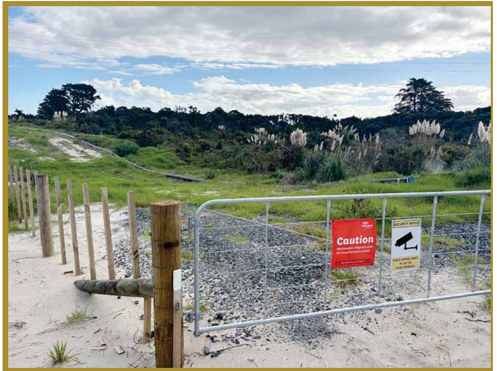
Council land at the end of Rama Rd. in Marden Point which is used for the disposal of treated wastewater from the Ruakaka Wastewater Treatment plant
