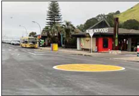
A simple painted on the road roundabout as suggested by the WRRRA.
