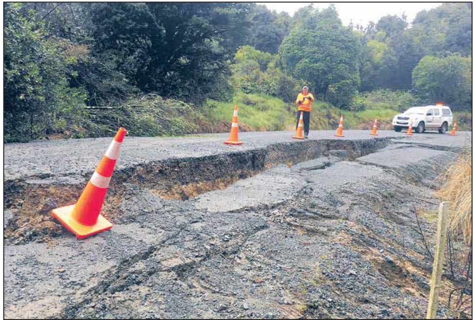
Towards the top of Helmsdale Rd. a section of road already coned off as it was beginning to slump prior to last weeks deluge was made worse with huge cracks widening and the road base moving further down the hillside,
