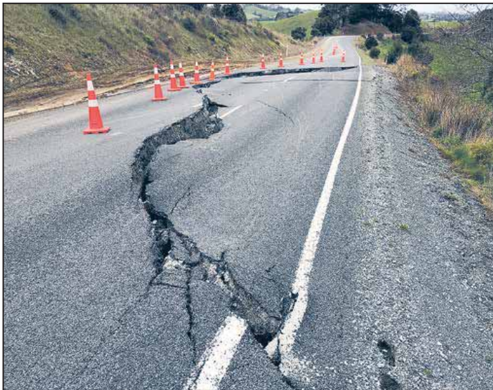
Subsidence at the top of the Shoemaker Rd. hill.
