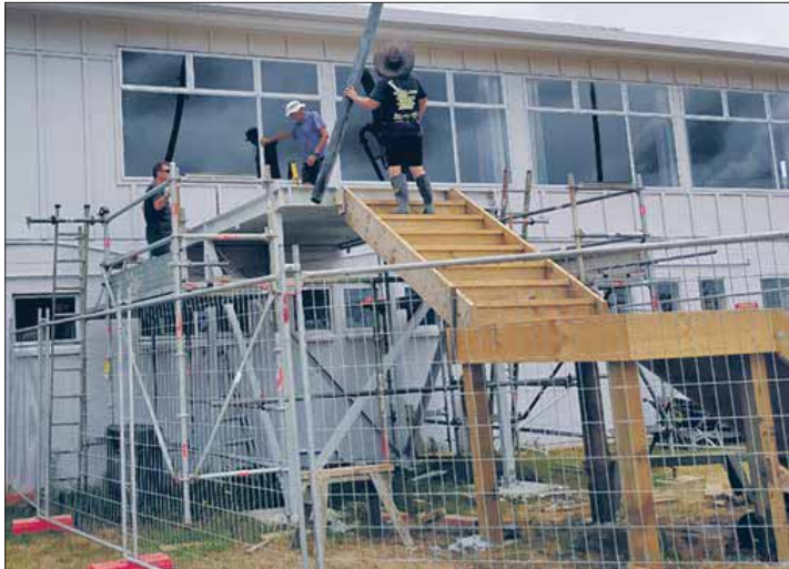
Builder Alan Mcintosh (centre) supervises the concrete pour on the new landing watched by Recreation Centre Committee Chairman Andreas Thirling.
