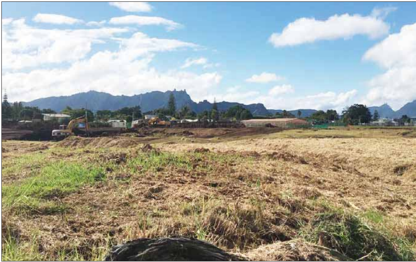
On Monday 22 April when this photograph was taken, it appeared that earthworks had already begun and no pond or wetland remained
