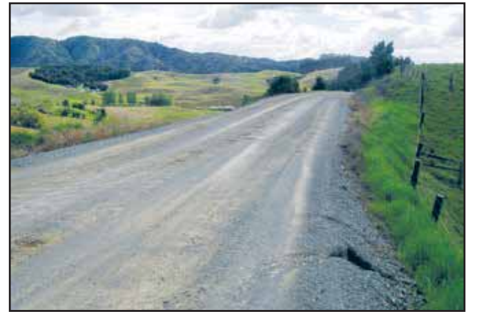
Pot holes,corrugations and mud on Brooks Rd.
