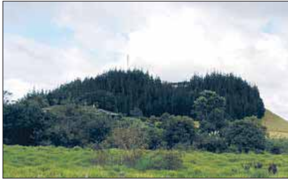
Sergeants Hill, the site of the Ruakaka water treatment plant
