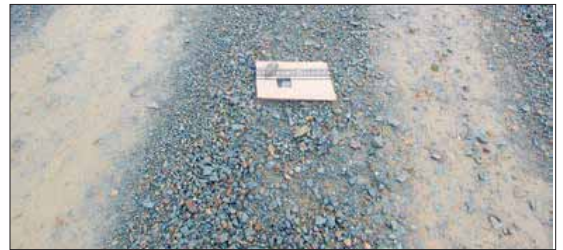
65mm gap metal has been puncturing the tyres of vehicles driving over it.
