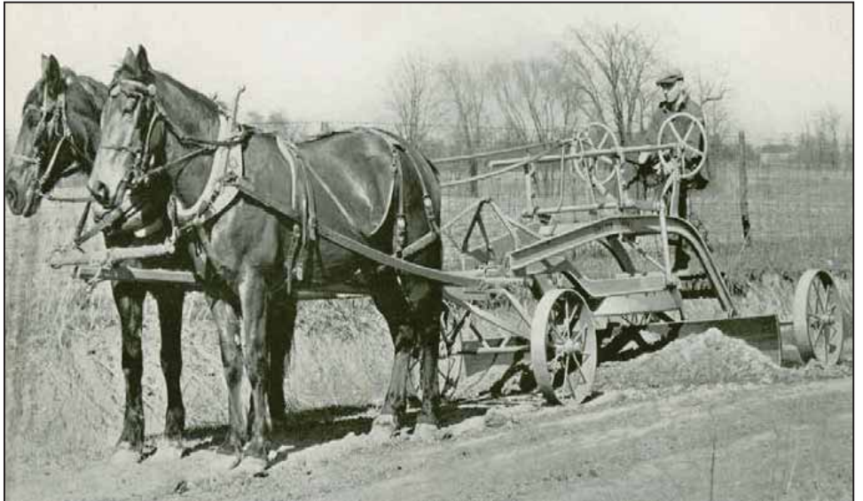
A horse drawn grader or scoop as used to construct the road over the Brynderwyn hills in the late 1930s
