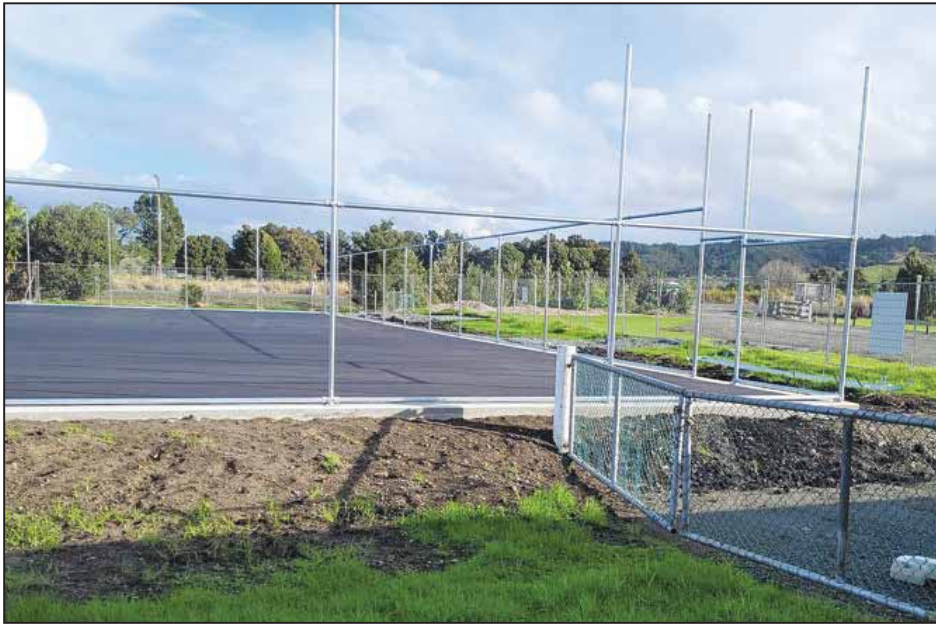
The new Takahiwai netball court
