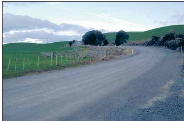
Applecross Rd. in Waipū has been rebuilt and has a layer of the new aggregate mix on the surface.
