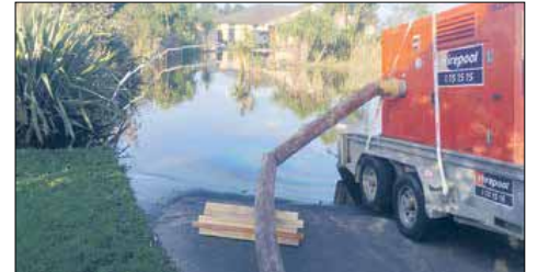
A pump was needed to bring down the water level at the Ruakākā Dune Lake after heavy July rain
