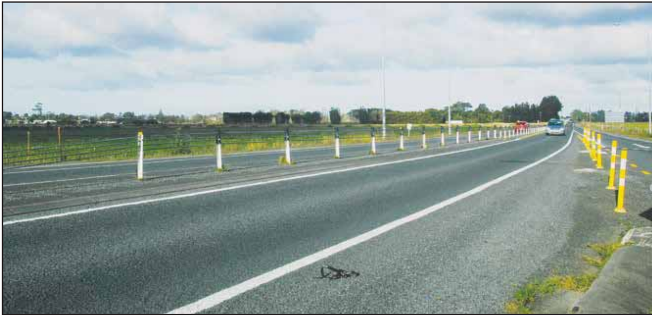
Safety barriers already installed on the highway at Ruakākā
