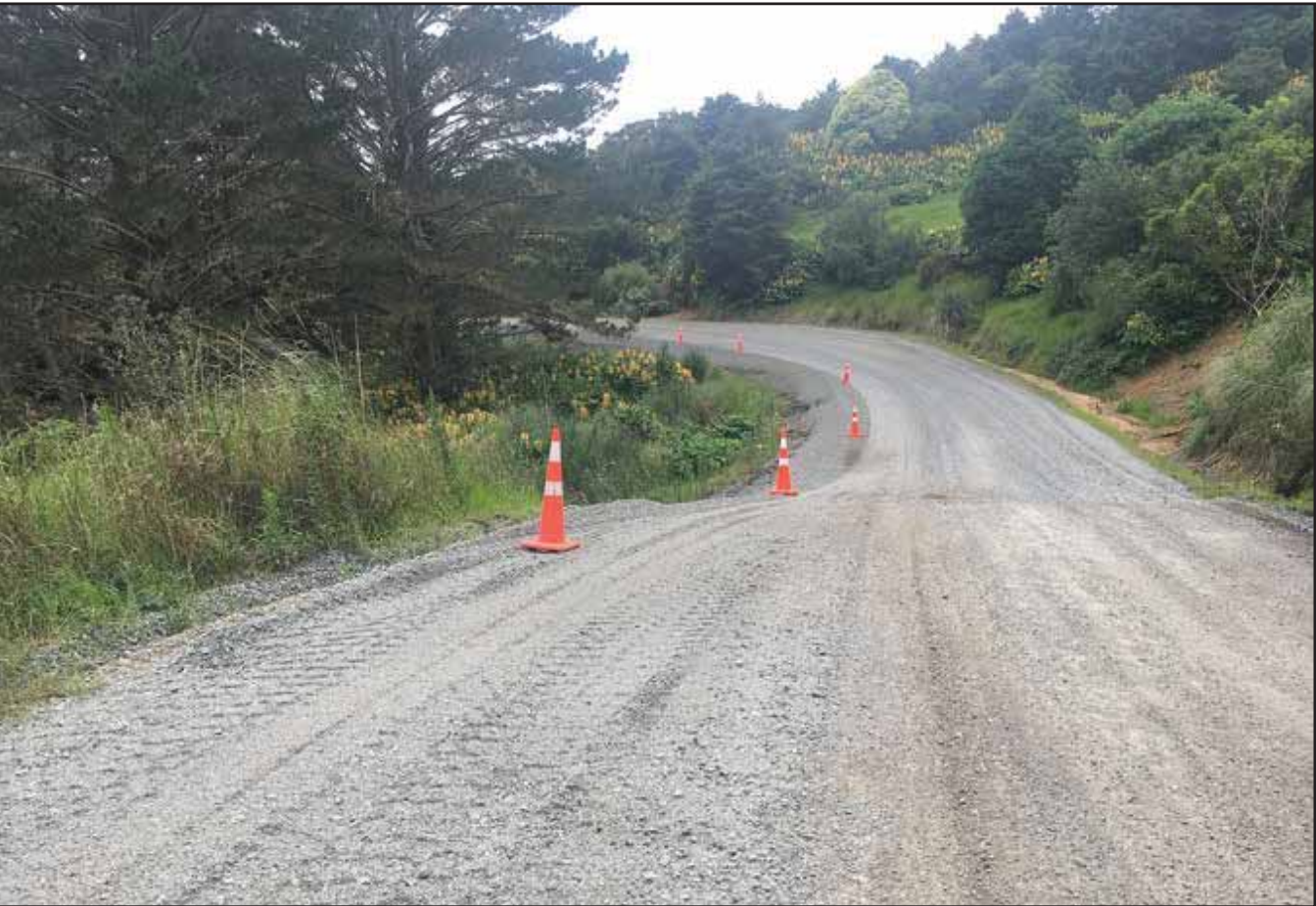
A section at the top of Helmsdale Rd where the road has slipped away to leave just a single lane
